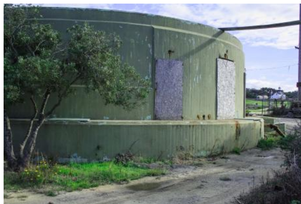
Pacific Grove Sewage Treatment Plant
