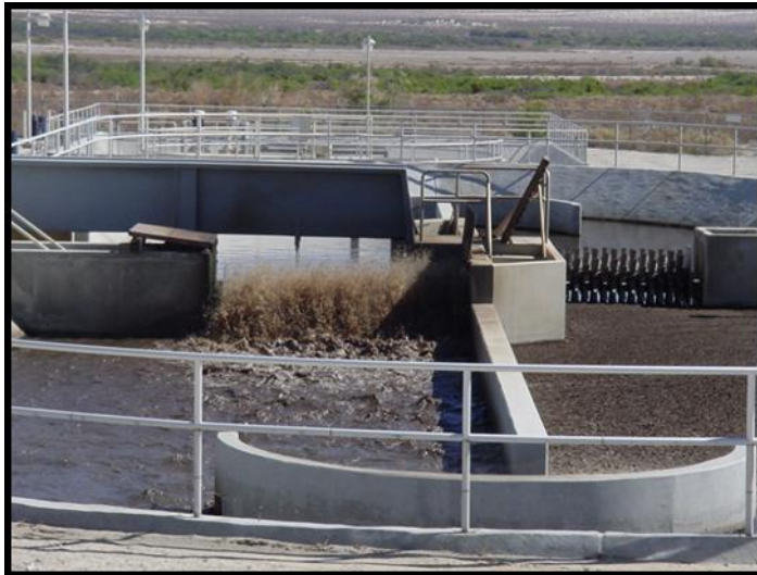
Wastewater Treatment Facility, Borrego Springs, CA
